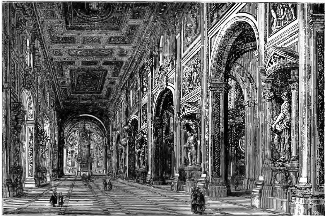
INTERIOR OF ST. JOHN LATERAN, ROME.
