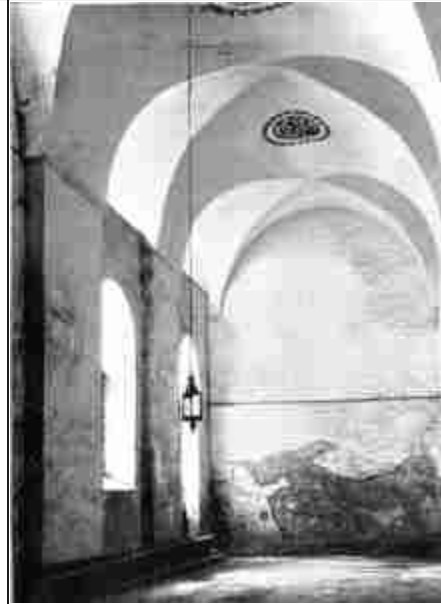
S. Saviour Pantokrator. Outer Narthex of the South Church, looking north.
