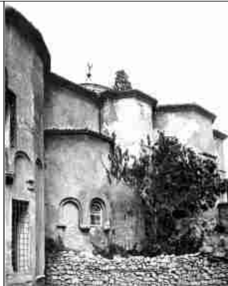
S. Mary Panachrantos. East End of the North Church.
