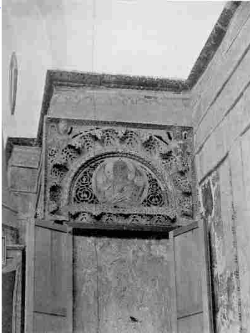
S. Saviour in the Chora. Eikon Frame on the south-eastern pier.
