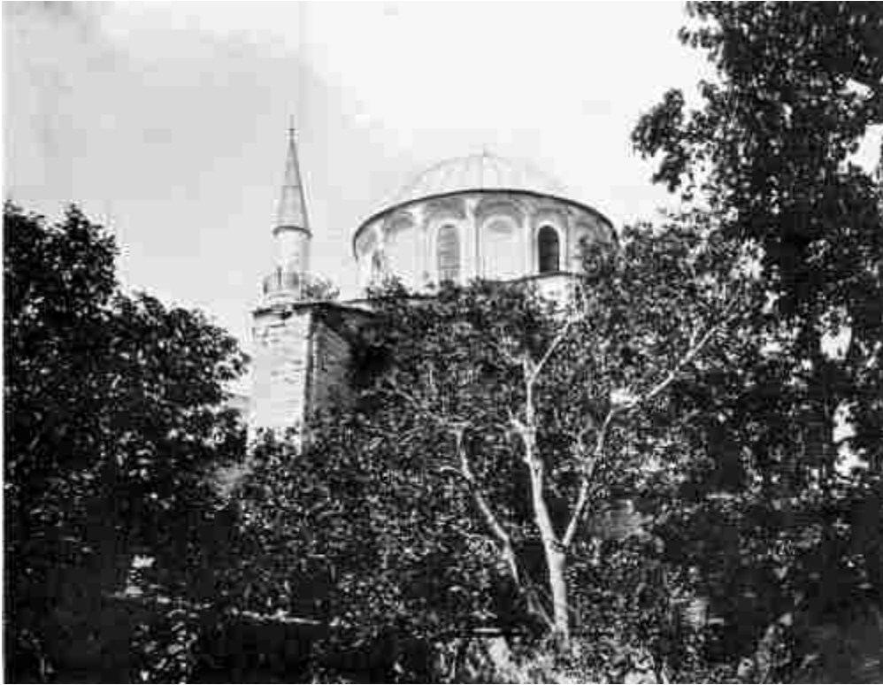
S. Saviour in the Chora, from the north-east.
