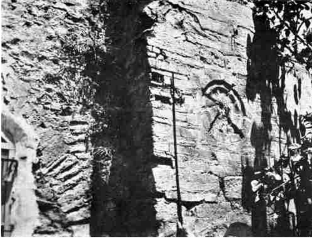
S. Saviour Pantepoptes. Exterior Decoration in Brick, on South Side
