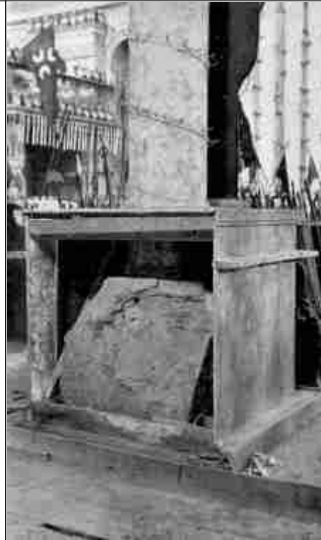
S. Irene. Base of Column in the South Aisle, seen from the South Aisle.
